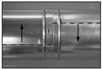
Figure 10.7 Rotate Seams for Disassembly
